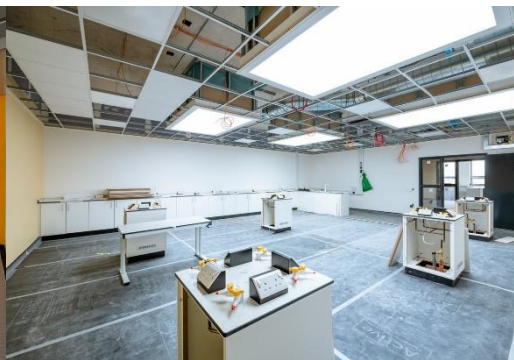
A science laboratory in progress up on the top floor.
